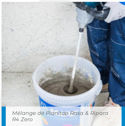
Application de Planitop Rasa & Ripara R4 Zero
